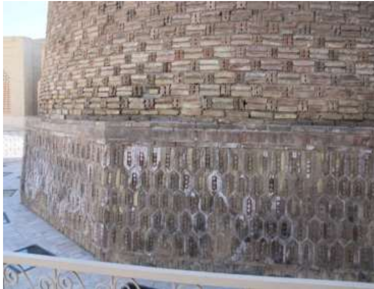
Figure 6. View of Salinity effect to the Kalyan Minaret fundament – Source: the authors
