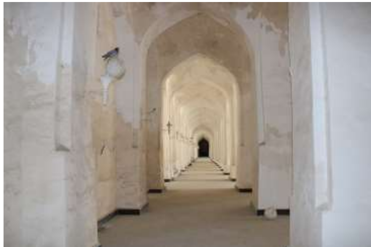
Figure 7. Kalyan Mosque, Right-hand pylons, affect of humidity to the walls and its decoration – Source: the authors
